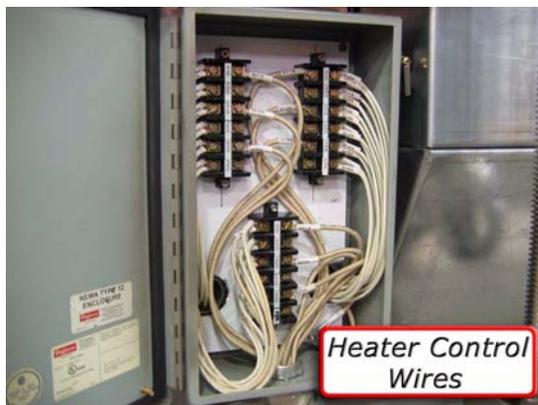
Figure 6.22: Heater Control Wires
